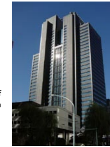
Shinjuku MYNDS Building
