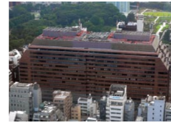
Shiba Park Building
